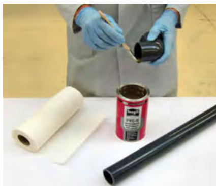
Applying the cement
