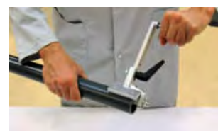
Chamfering the pipe
